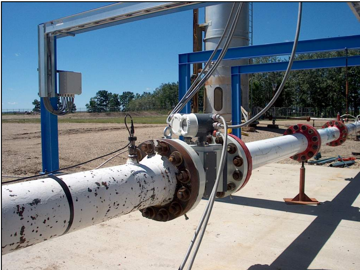
Figure 18 – Meter Pulsation Testing at Nova’s Didsbury Facility
