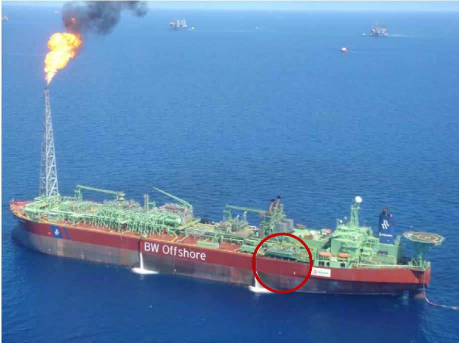
Fig. 6 The Meter Skid on a Vessel
