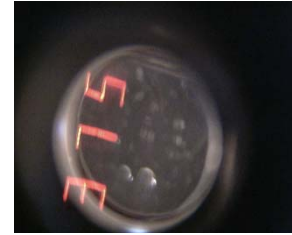
Large amount of Hydrocarbon Liquids on Mirror
