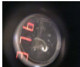
Glycol & Liquid Hydrocarbons On Mirror
