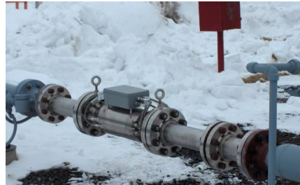
Figure 4. Use of Multiple Paths to Improve the Accuracy of Volumetric Measurement.
