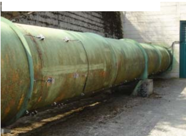
Figure 9. Multipath Clamp-On System Providing Turbine Output Control.
