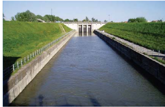
Figure 11. An Open Channel using Transit Time Technology to Measure Flow.
