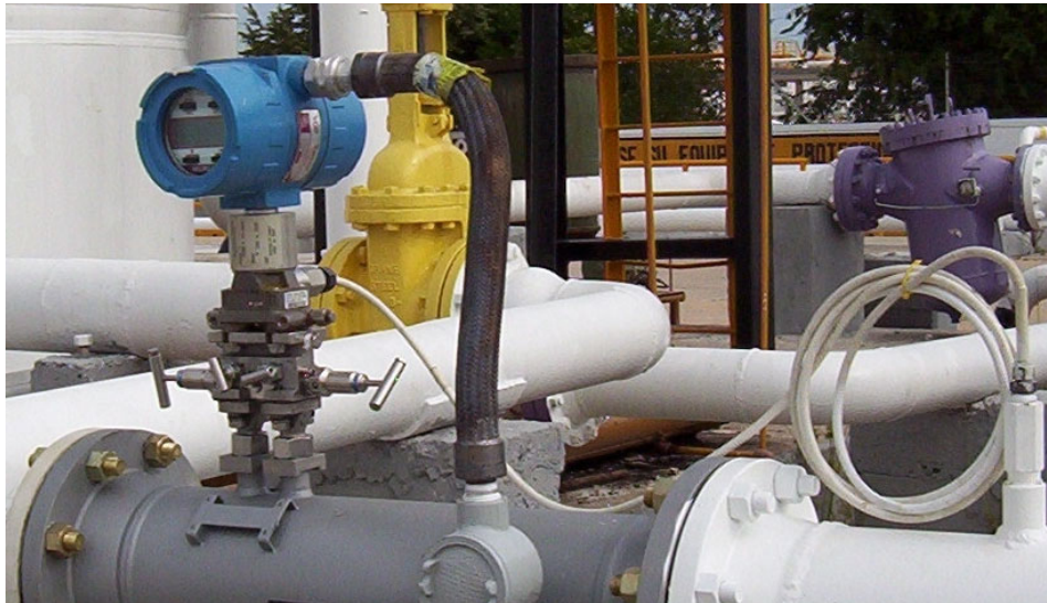
Figure 6.0 Typical Remote Mounted System
